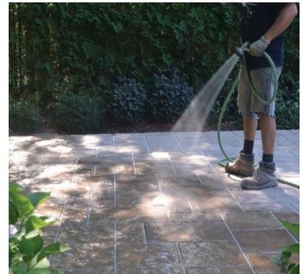
**B** • Repeat the showering of the patio surface as above for a second and third time, waiting 3 to 4 minutes between each shower. However, stop watering when no more water will soak into the joints. If the work is being done on a hot summer day, avoid spraying large areas at a time, as they will dry unevenly.
